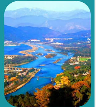
Visit Dujiangyan Irrigation System
